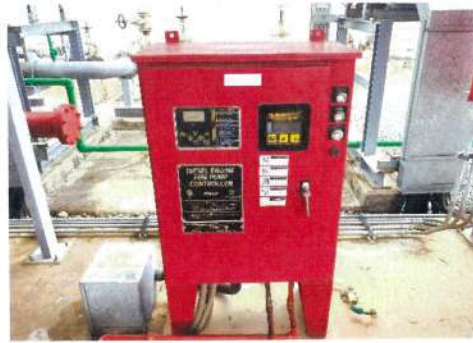
Fire pump controller
