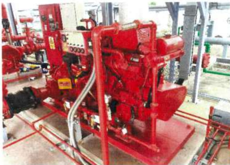
Diesel engine fire pump
