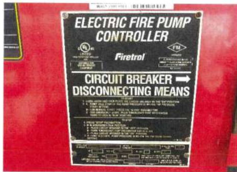
Control panel certified name plate
