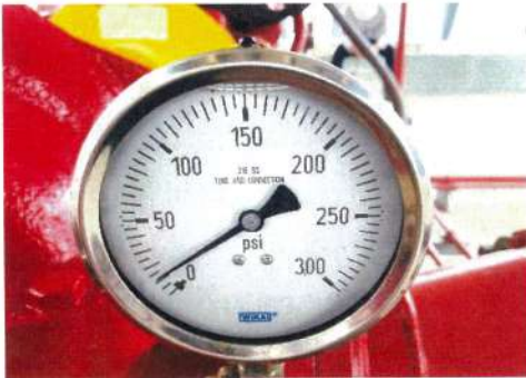
Discharge pressure gauge
