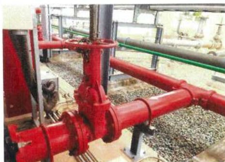
Suction isolate valve opened
