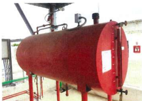
Diesel fuel storage tank
